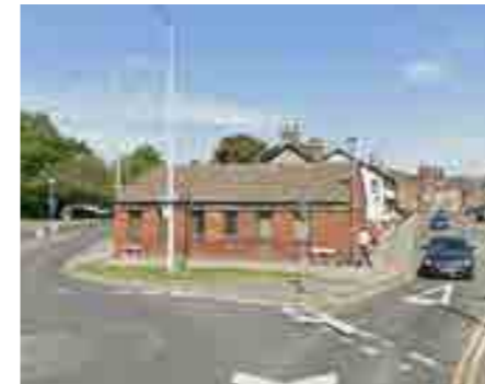
Southern gateway to the town centre - credit Google Images
